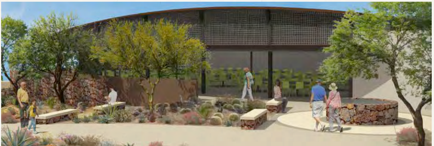
Pavilion front showing adjustable weather panels.
