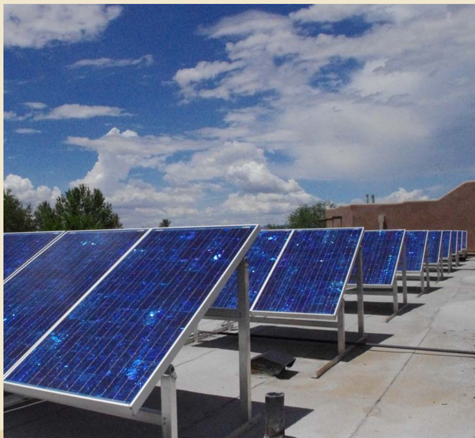
Solar panels atop Tohono Chul's Education Center provide about 5,000 kilowatt-hours of energy annually.
